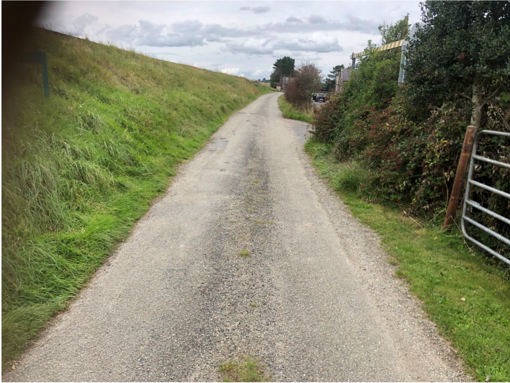
Photograph No.1: View of Existing Roadway taken in or around CH00 looking west.
