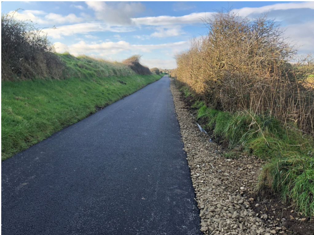
Photograph No.4: Emergency remedial works carried out in 2023.
