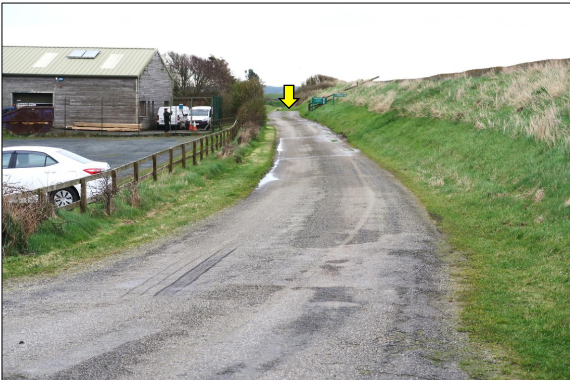
Plate 12. The Visitor Centre Car Park and the reserve workshop and storage shed (left) and the end point of the proposed resurfacing works (arrowed)
